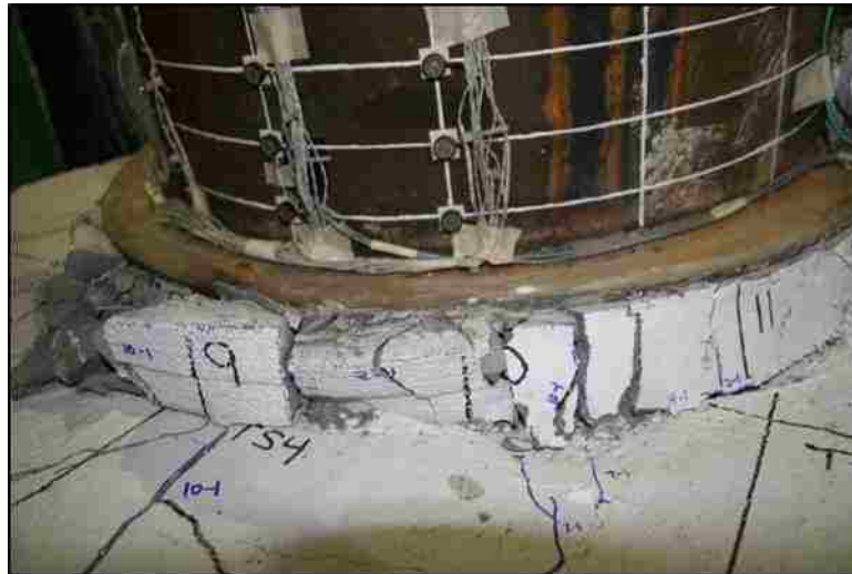
Figure 5.34: WRC South soffit damage at 11.47% drift South
