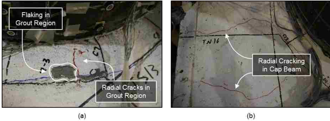
Figure 5.6: EMB80 Radial cracking at 1.45% drift in (a) grout region, and (b) cap beam
