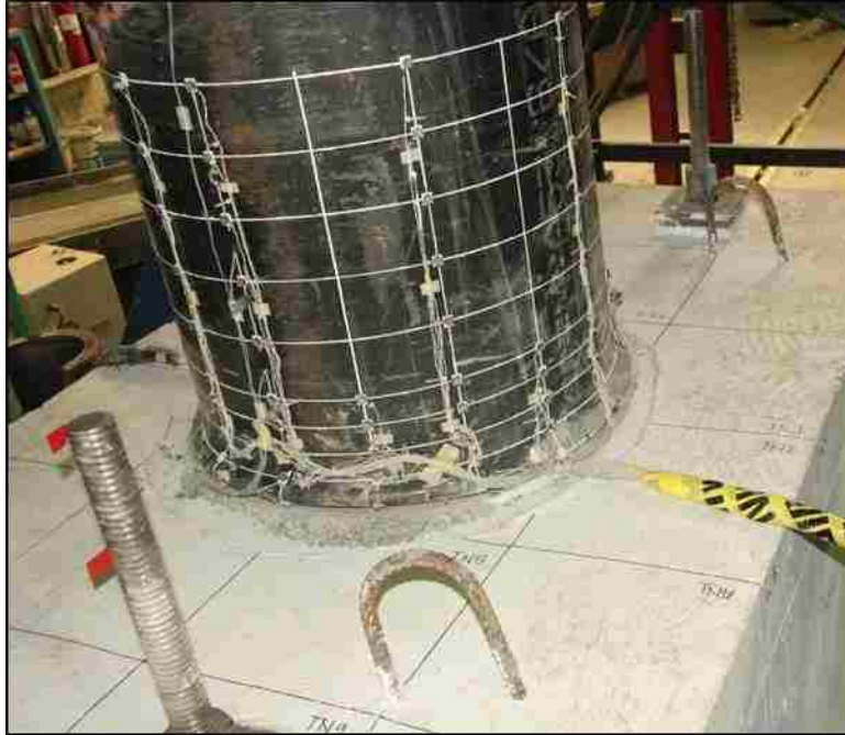
Figure 5.73: EMB96 Specimen damage at termination of test
