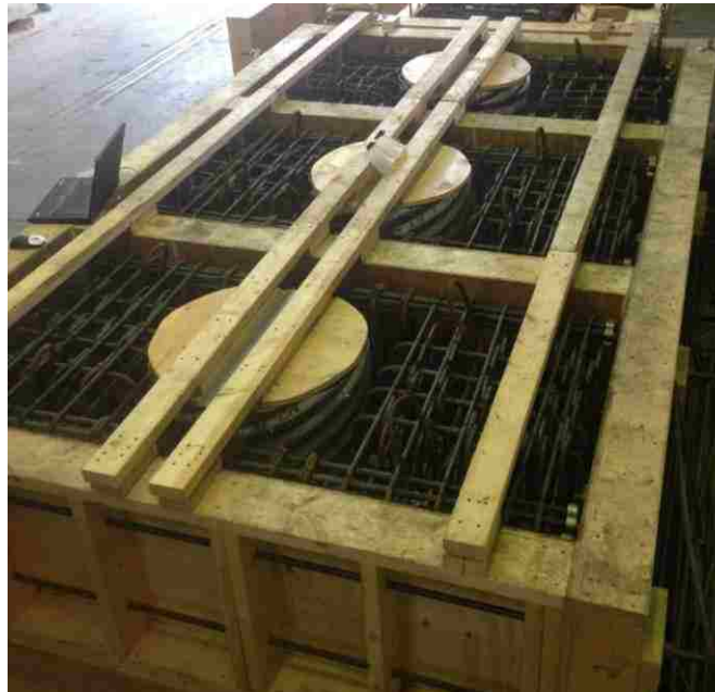
Figure 4.7: Cap Beam Reinforcing and Formwork
