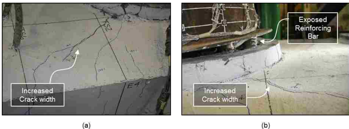
Figure 5.45: WRCUB South (a) cap beam cracking, and (b) exposed reinforcing bar at 8.19% drift North
