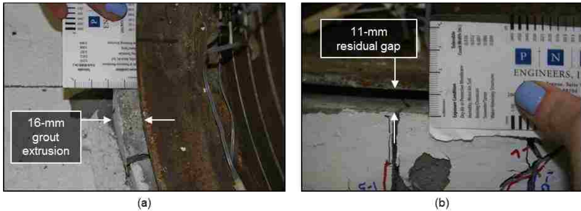
Figure 5.44: WRCUB (a) grout extrusion, and (b) residual soffit-flange opening after 13th cycle level
