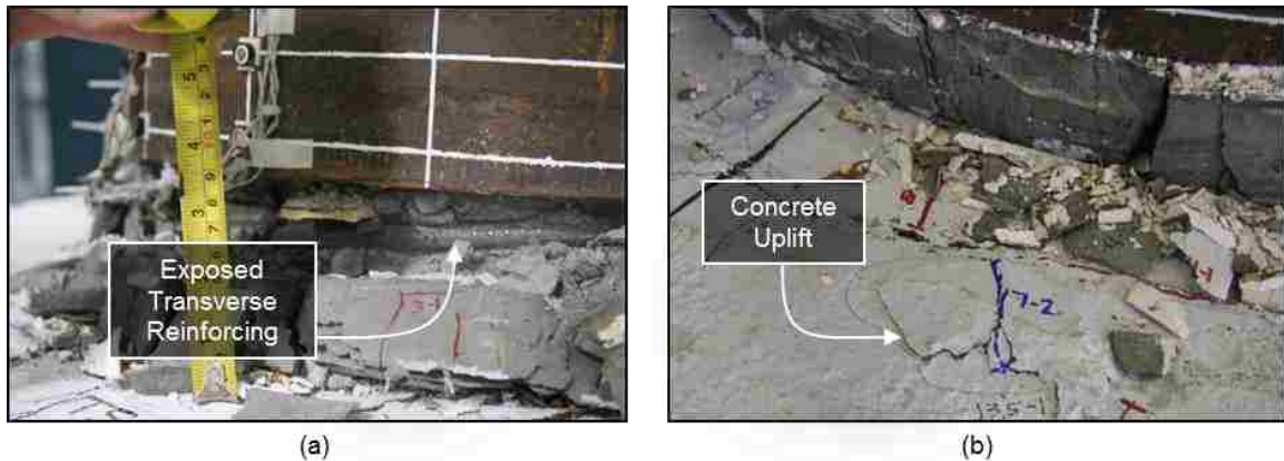
Figure 5.58: WRC (a) South transverse reinforcing, and (b) North concrete uplift at 8.15% drift
