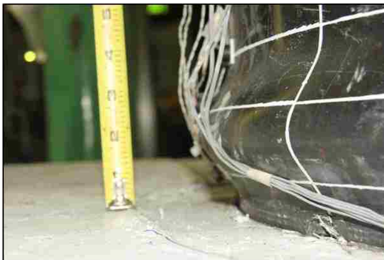
Figure 5.72: EMB96 South local buckling after 14 th load set
