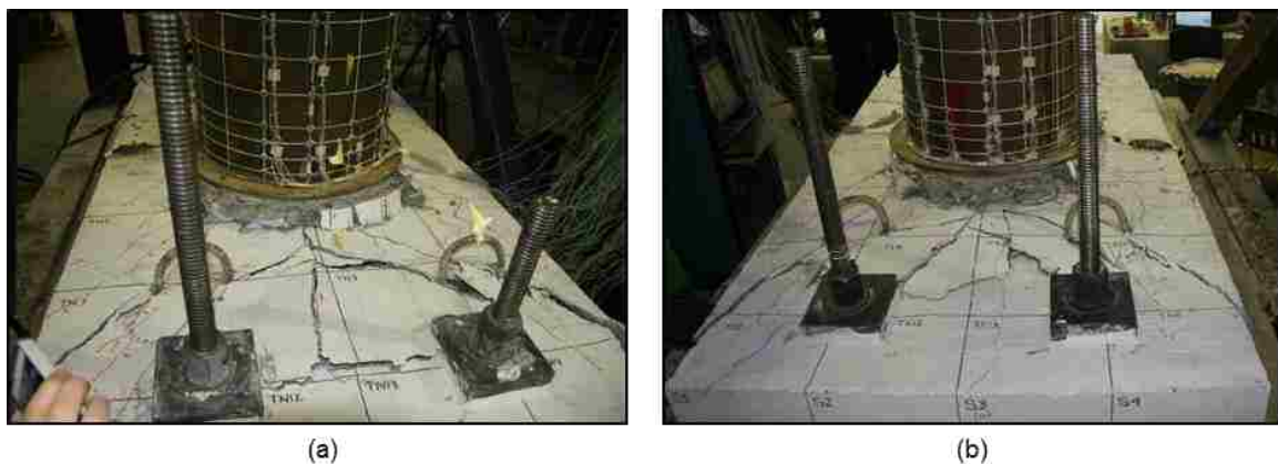
Figure 5.36: WRC (a) North, and (b) South cap beam damage after test termination
